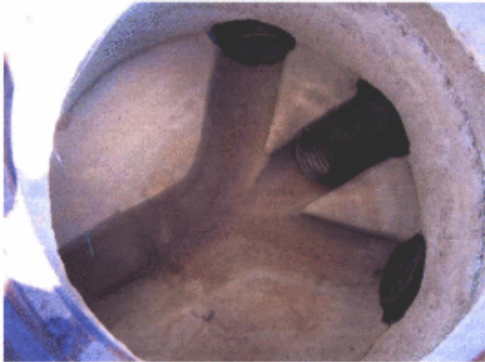
Photo 13 Manhole/Drain E at south west corner of cap 5/23/07
