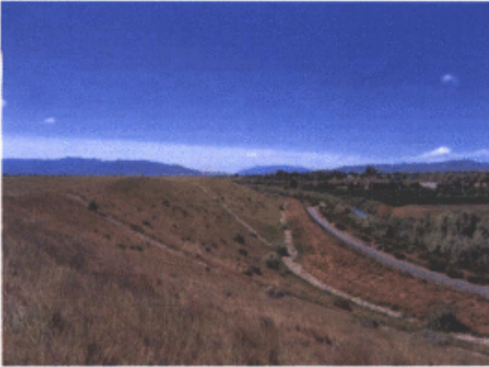
Photo 19 View to the south of the caps west slope 5/23/07
