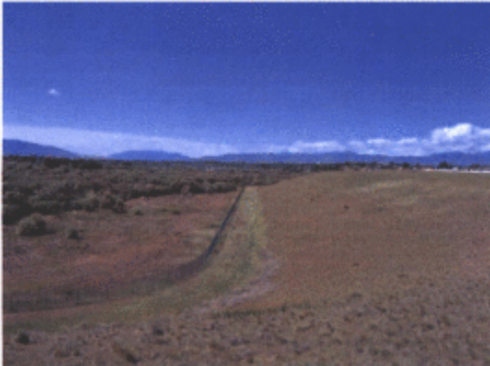
Photo 21 View to the south of the caps south east slope 5/23/07
