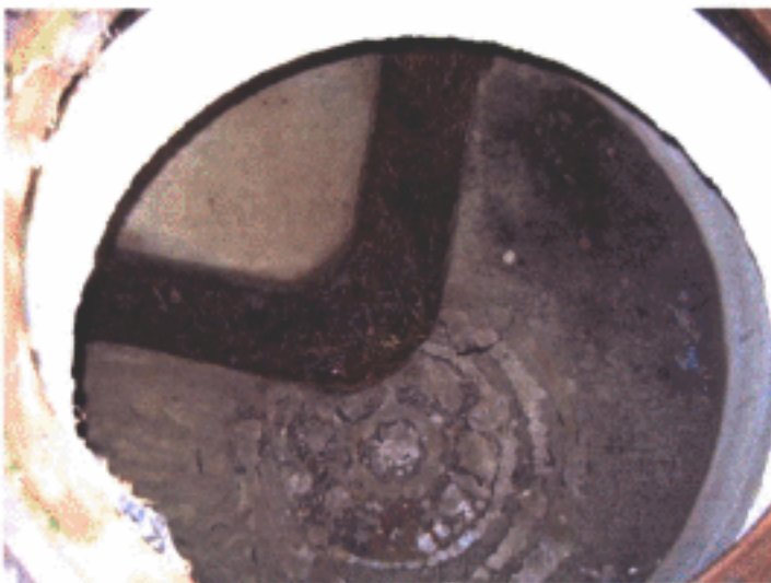
Photo 11 Interceptor Trench Manhole/Drain G 5/23/07
