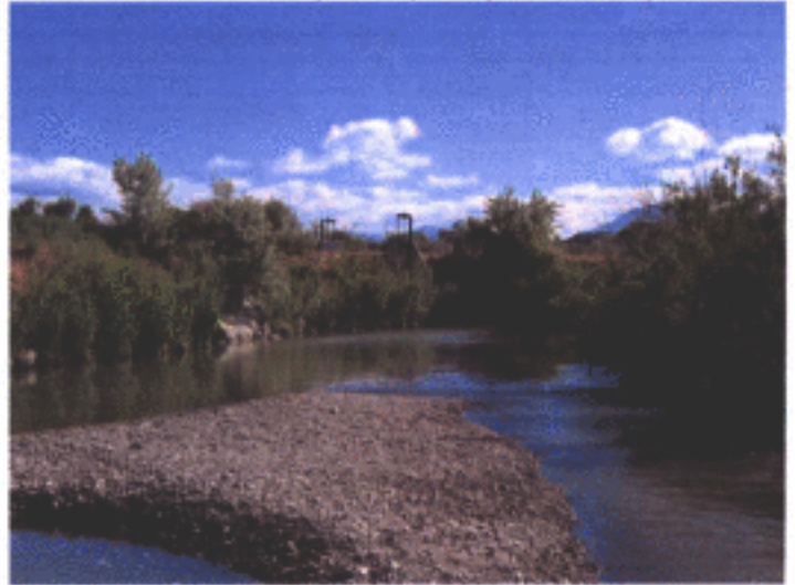
Photo 8 Jordan River Erosion Area E 5/23/07
