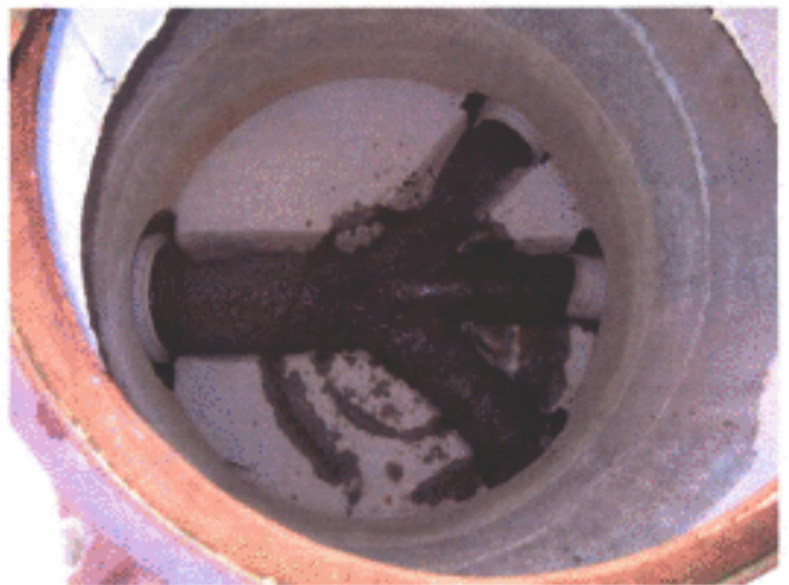
Photo 12 Manhole/Drain F at south central corner of the cap 5/23/07
