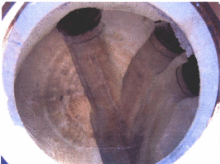
Photo 17 Manhole/Drain A at the base of the caps west slope 5/23/07
