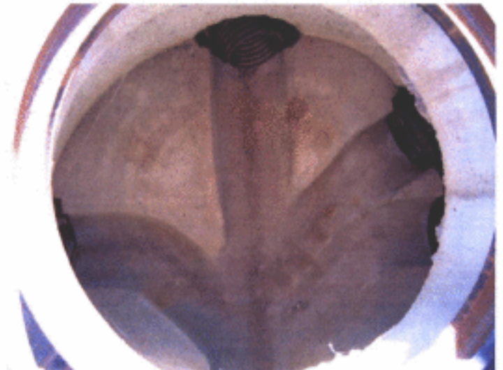
Photo 16 Manhole/Drain B at the base of the caps west slope 5/23/07
